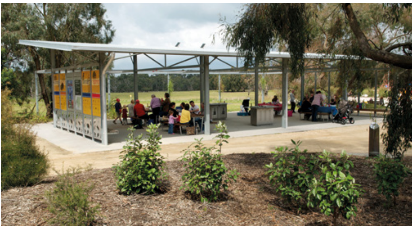
Figure 27 Shelter pavilion and barbecues at the Woodland Picnic Area
